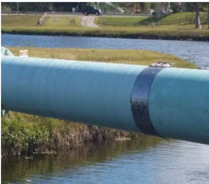
Figure 4 - Repair to 24" DIP
