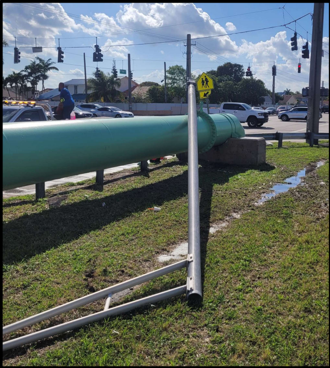
Figure 2 - Picture of Car Accident which caused Spill Event on February 19, 2022
