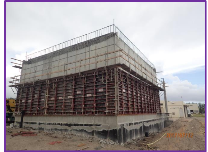
Site 2 Bldg under construction
